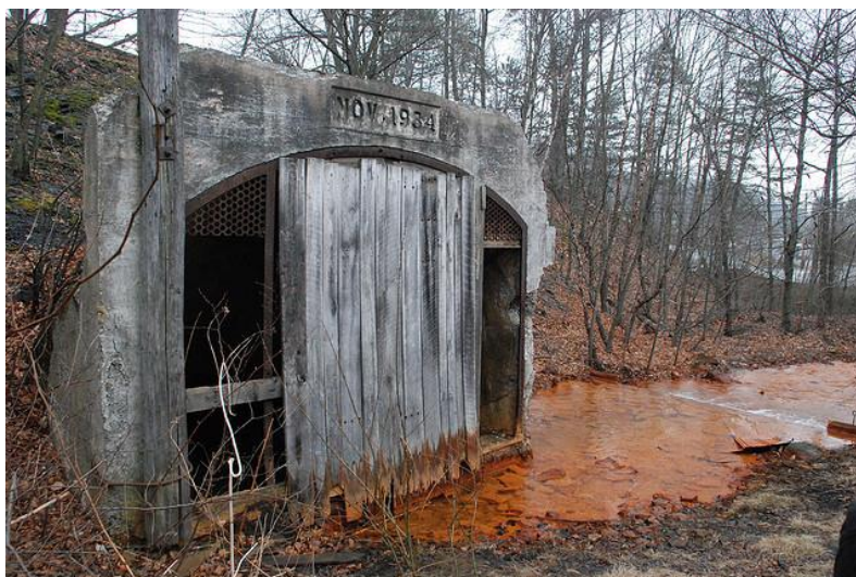
Figure 1: An example of acid mine drainage flowing into Shamokin Creek. Notice the red-orange color of the water.
